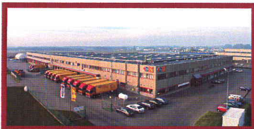
HBH Offices Poznań, Poland
